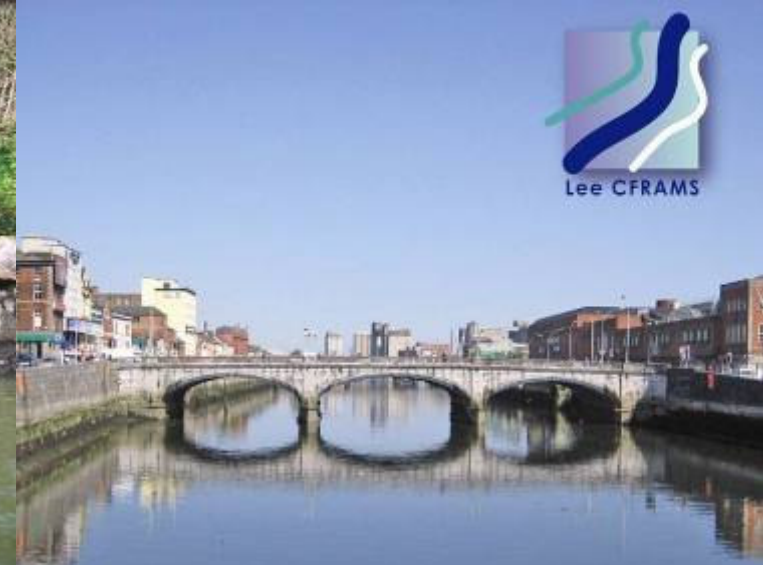
St. Patrick's Bridge in Cork City
